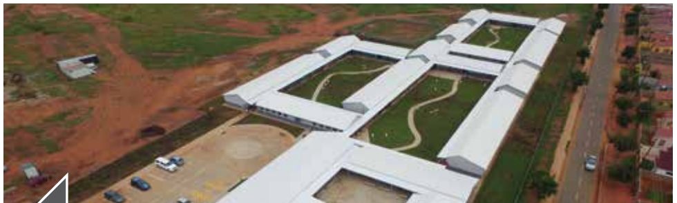
Sale of a 1 000 student school, using alternative building technology compliant to SANS
