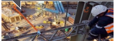
SGB Cape: QuikDeck platform being assembled in the air by a specially trained Waco employee.
