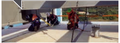
SGB Cape: Vulindlela Project where the QuikDeck team complete the QuikDeck Suspended Access System.
