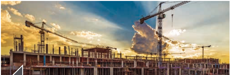
Form-Scaff: Mall of Africa, Midrand.
